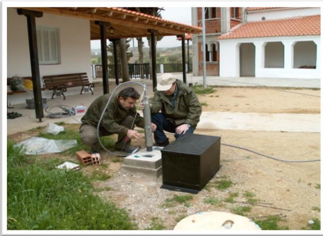
Photo 1: Location of the PRO_033 borehole
