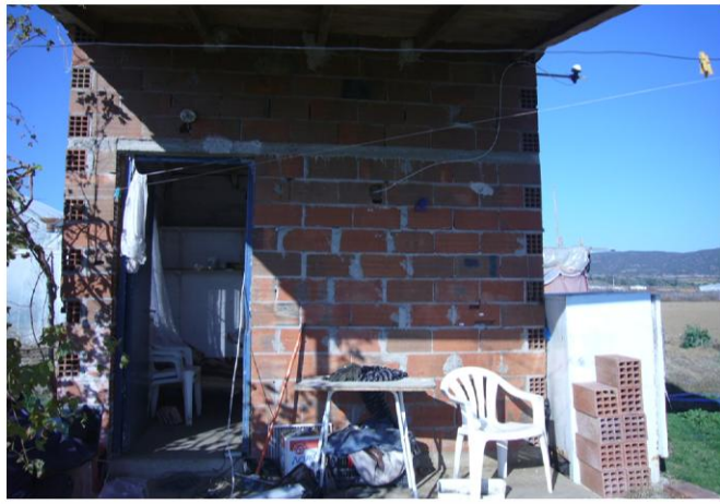
Photo 1: Outside view of the hosting building
