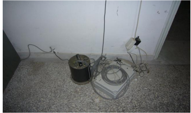
Photo 2: The STC station
