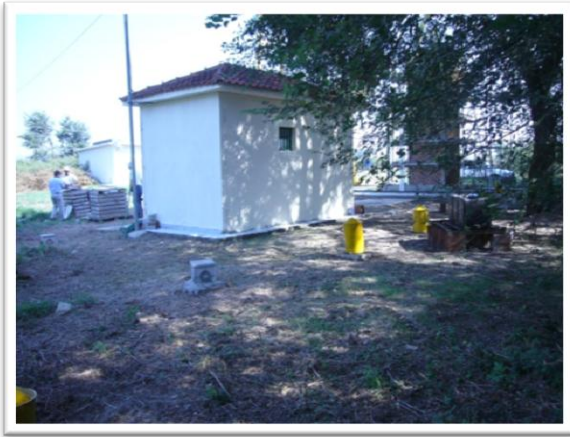
Photo 1: Outside view of the hosting building
