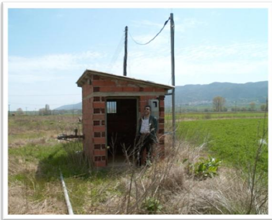
Photo 1: Outside view of the shelter
