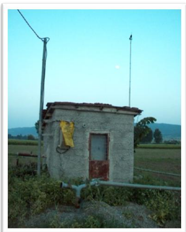
Photo 1: Outside view of the hosting shelter
