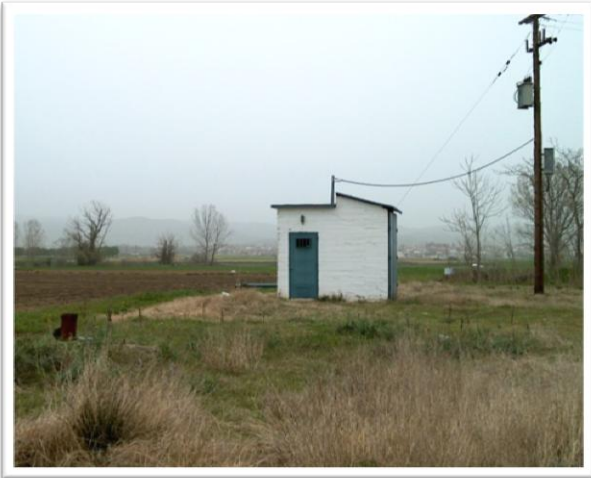
Photo 1: Outside view of the hosting shelter
