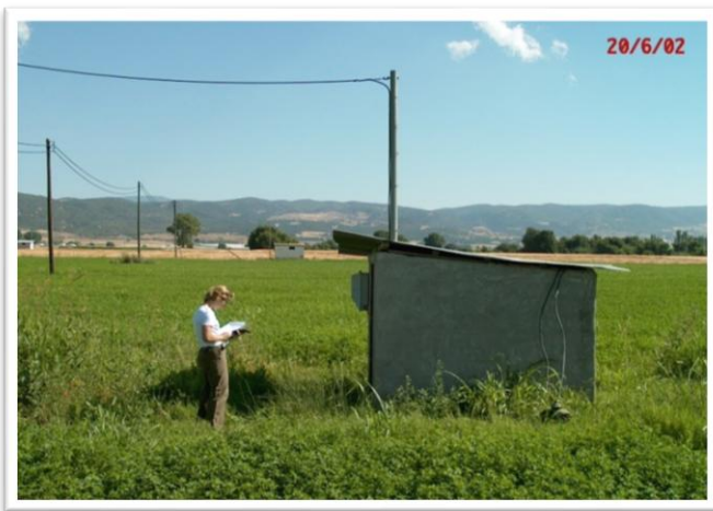
Photo 1: Outside view of the hosting building
