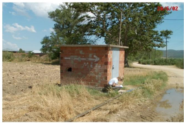
Photo 1: Outside view of the hosting structure
