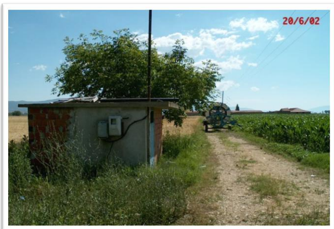
Photo 1: Outside view of the hosting structure
